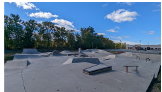
Skate Park - View Looking Southwest
