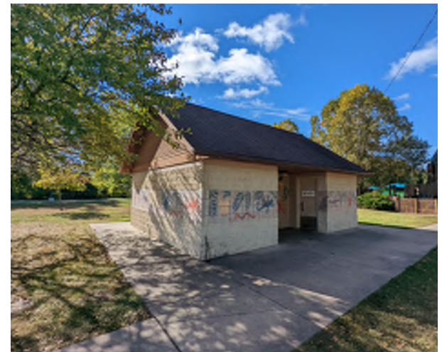
Existing Restroom Facility
