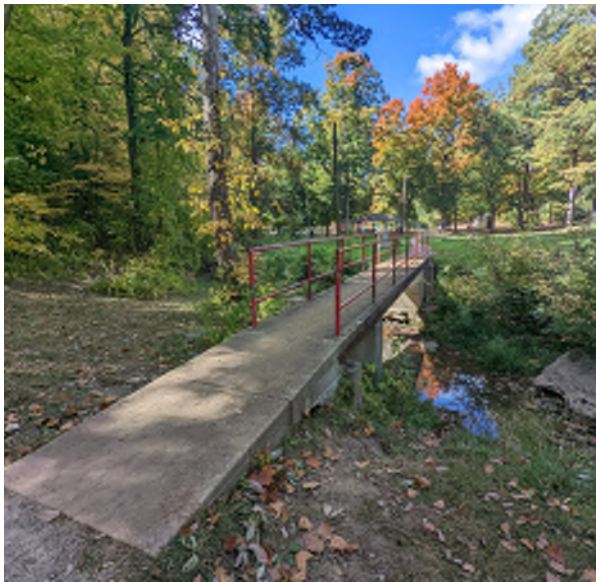
Bridge at Maconaquah Park
