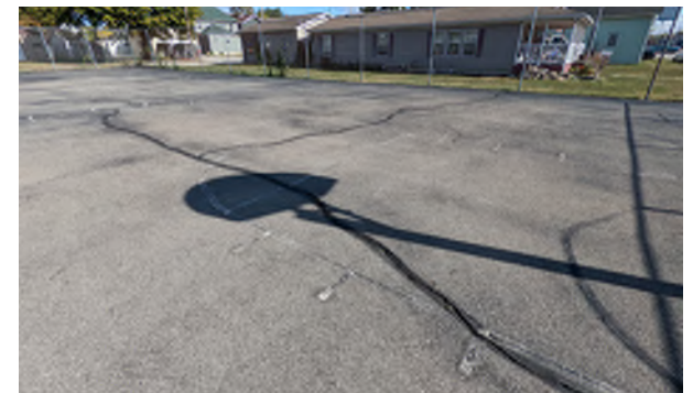
Court Asphalt Surface
