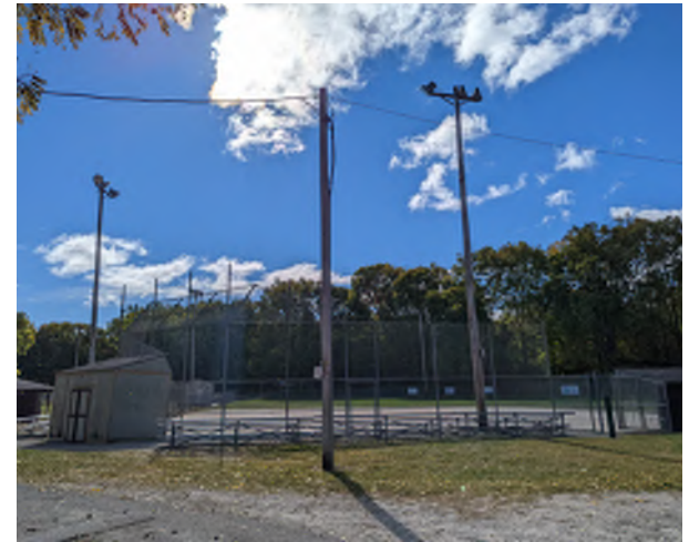
Existing Fields and Lighting
