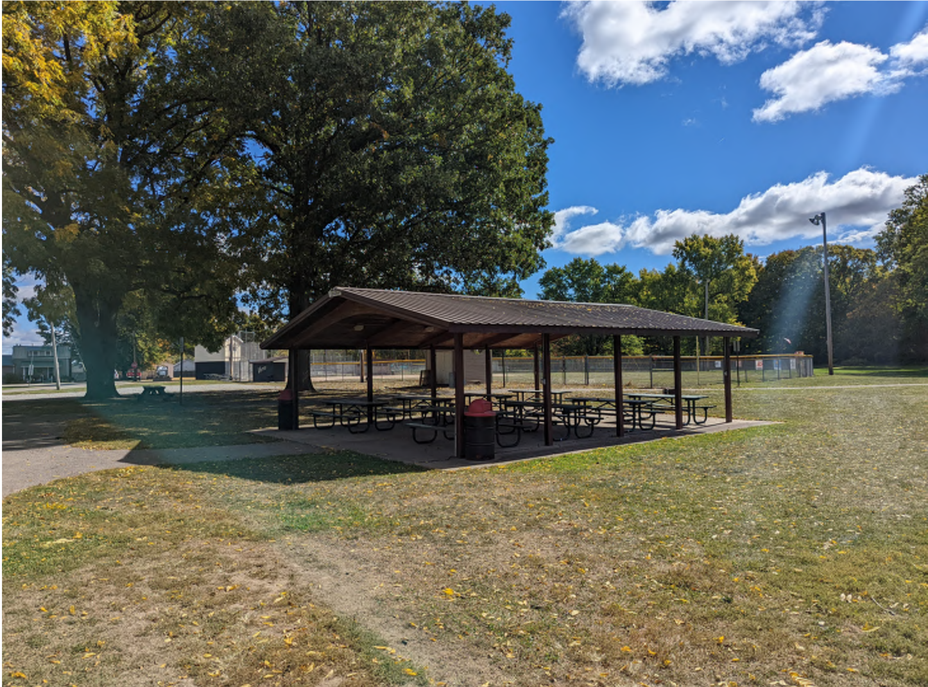
Shelter at West City Park
