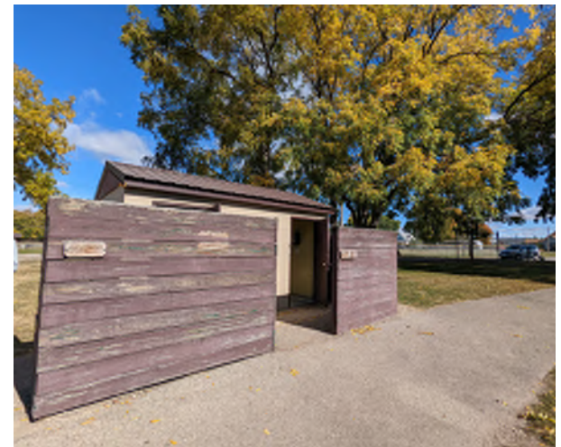
Existing Restroom Facilities
